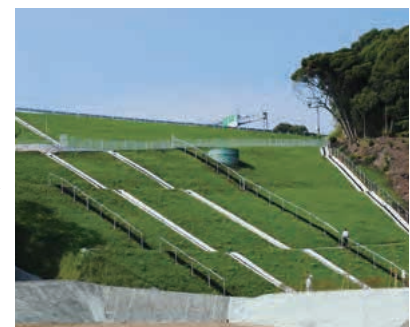
After full restoration (July 2010)
