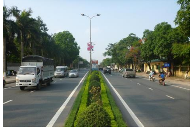
Pic 2: Improved section of existing National Highway No.1
